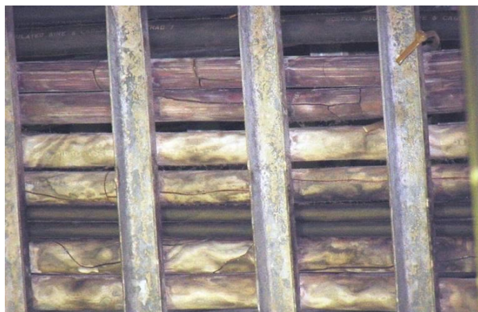
Pic 2 Aged cables in power station showing cracking.
