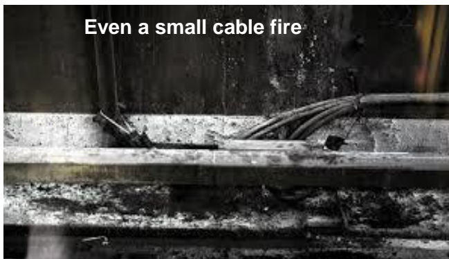
Singapore MRT 2013 - Newton Underground Station. Cable overloaded and caught
